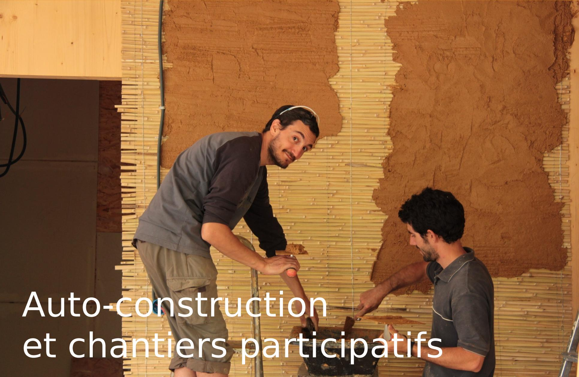
A photograph showing two men engaged in a construction project. They are working on a wall that is partially covered with a thick, brown, textured material, likely mud plaster, which is applied over a base of horizontal bamboo strips. The man on the left is leaning over a metal frame, using a tool to work on the plaster. The man on the right is standing and also working on the plaster. The background shows more of the wall and some wooden panels on the left.
